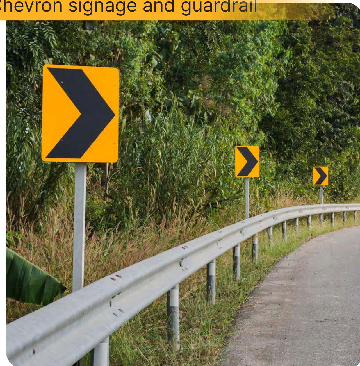
Chevron signage and guardrail
