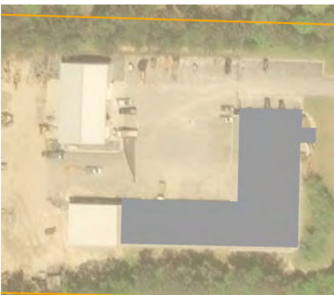
Figure 41. Pyles Plumbing Parcel
