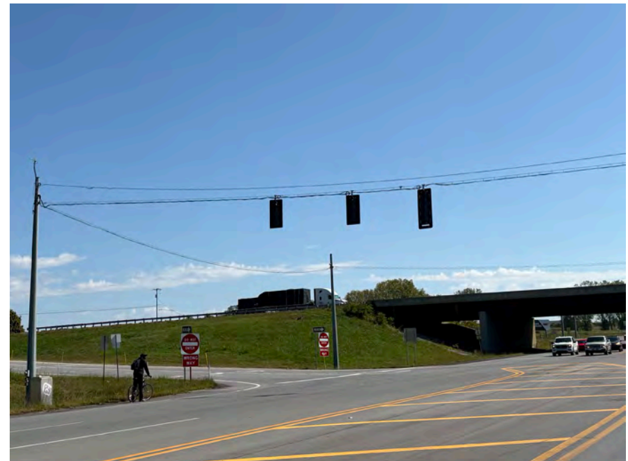
Figure 15. Bicyclist crossing the I-65 interchange on Scottsville Road (KY 100) in Franklin
