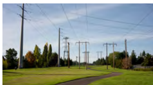
A trail following an overhead utility corridor.
