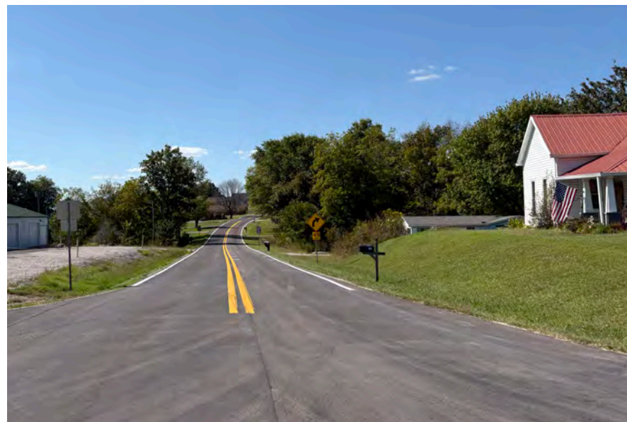
Rural roadway in Barren County
