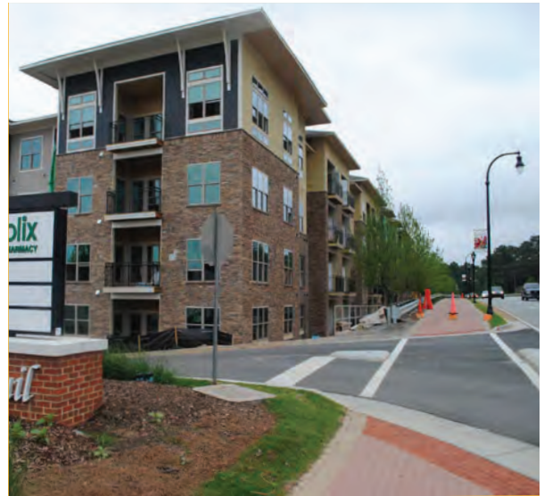
Trails near homes and destinations like grocery stores make walking and biking more viable options
